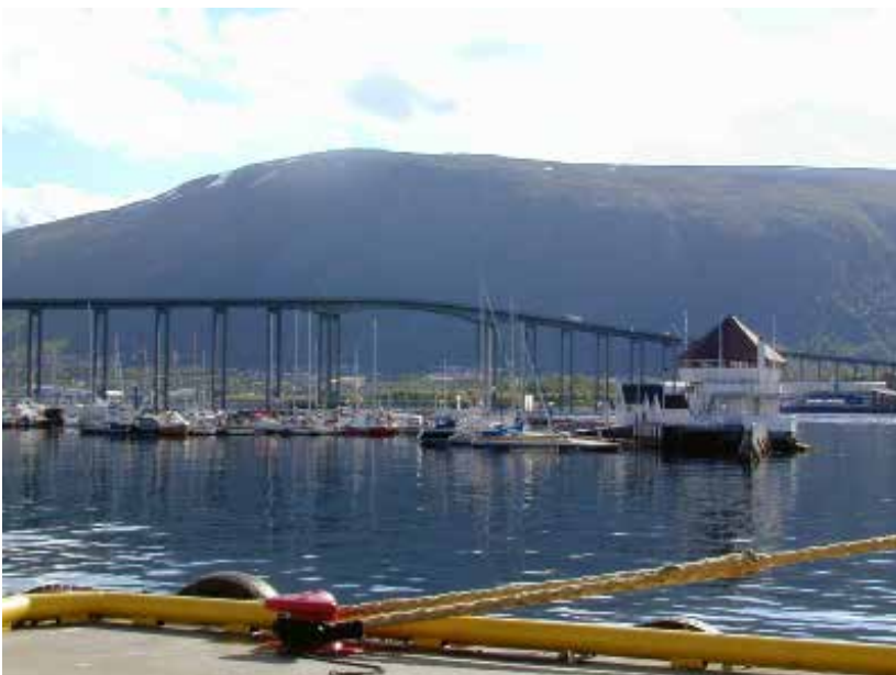
Tromsbrua Bridge, connecting Tromsøya to the Mainland (Randi M Solhaug)
