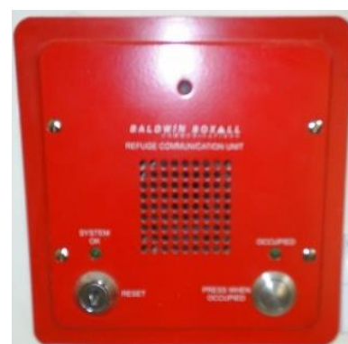
Braint Refuge Point: Found by the lift (not ground floor)
