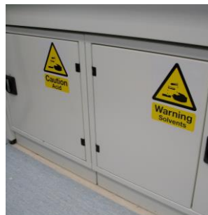
Ventilated Acid and Solvents Store
