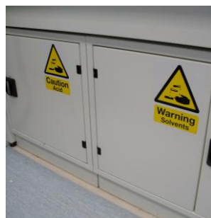
Ventilated Acid and Solvents Store
