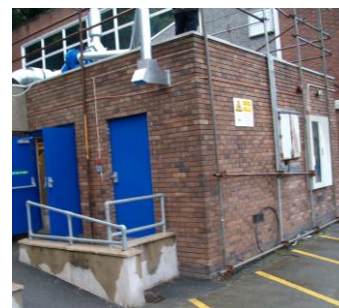
External bulk Chemical Store
