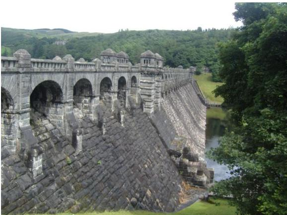
The dam construction started in 1881 and was completed seven years later in 1888. It was the first large stone-built dam in the United Kingdom, and is built partly out of blocks of Welsh slate 144 ft from the bottom of the valley, 128 ft thick at the base, 1,171 ft long with a road bridge running along the top.
