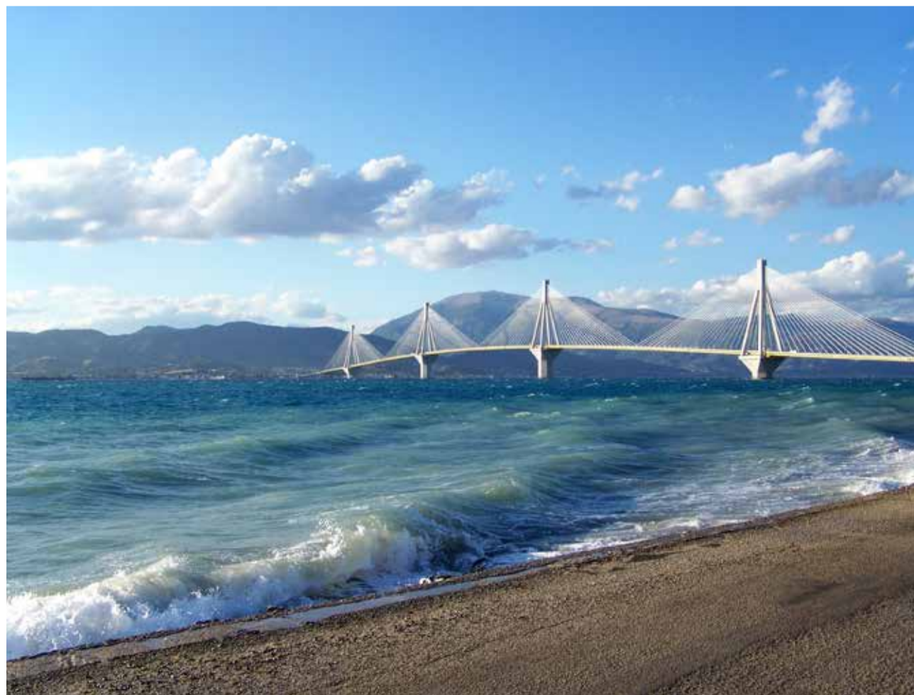
Bridge over Gulf of Corinth
