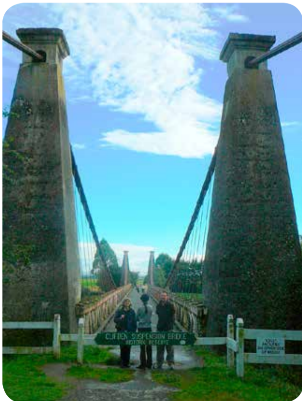
Jenny, with our son Ben and daughter Rosi, by the stone-clad concrete pillars of the Clifden Suspension Bridge.
