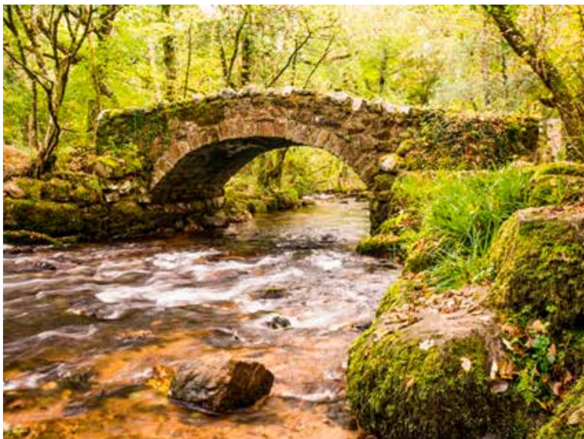
Bridge over the River Bovey
