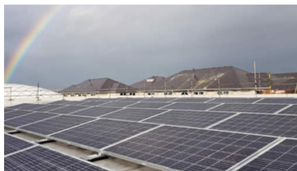
Solar Photovoltaic Panels installed on the roof of Canolfan Brailsford
